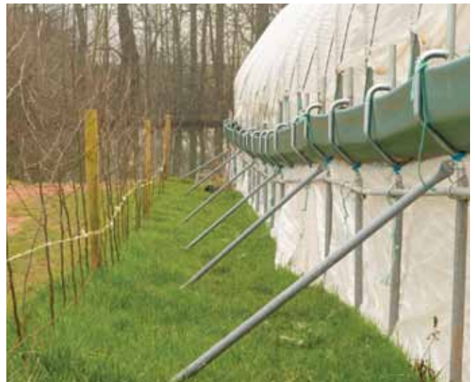
Harvested rainwater is collected from polytunnels in the guttering shown and then collected in the lined reservoir to be used for irrigation
