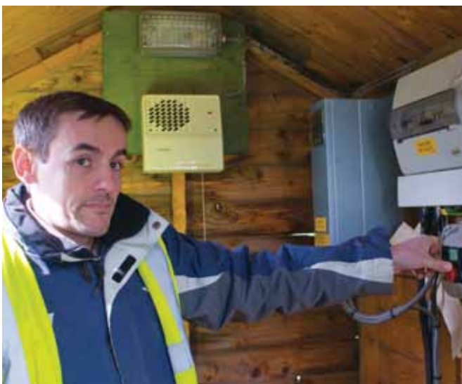
You need to think about how much energy a new system may use
